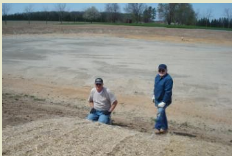
Mike & John lay straw mat on seeded dike
